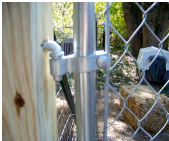
Figure 35. Top lag screw with hinge
