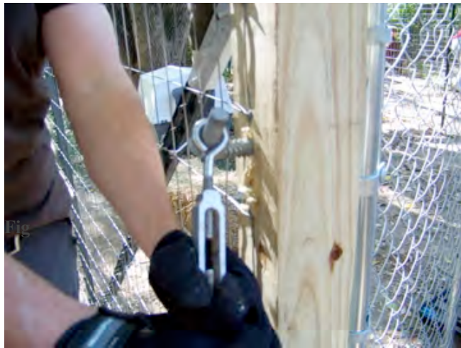
Figure 34. Screw in the lag screws
