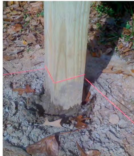
Figures 4a and 4b. String for aligning t-posts and String wrapped around a corner post
