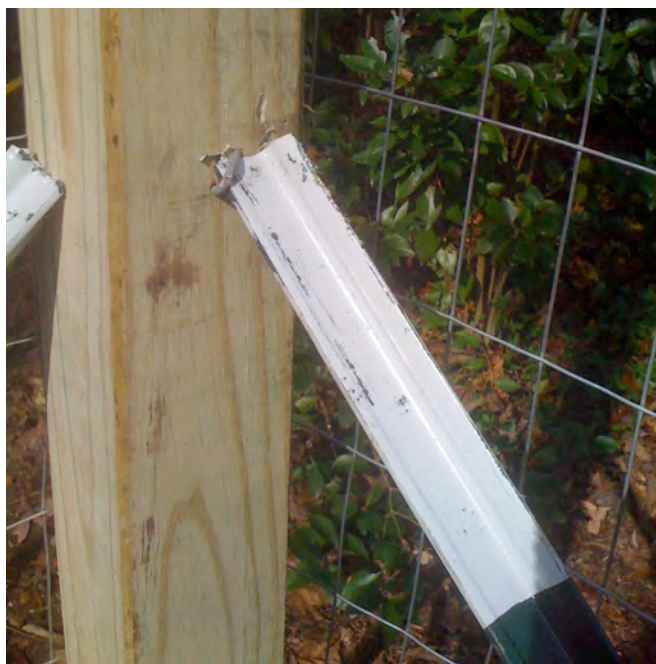
Figure 7b. Staple helping to secure corner support post.
