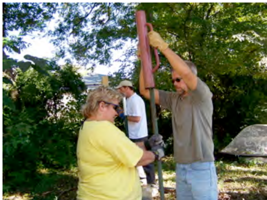
Figures 14 & 15. Driving the t-posts
