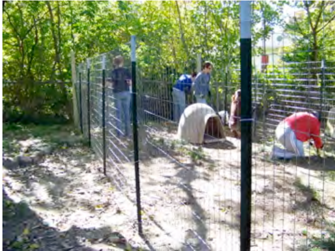
Figure 13. Placement of vertical t-posts
