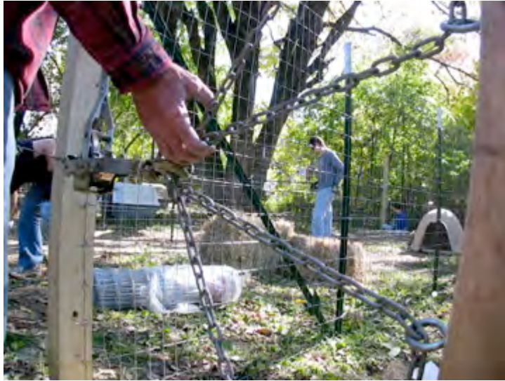
Figure 24. Attach the come-along to the fence puller
