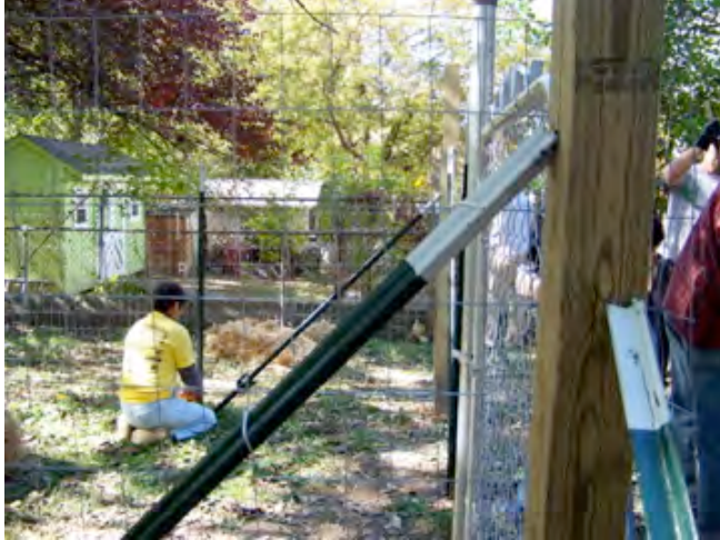
Figure 5. Placement of diagonal support
