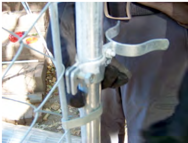
Figure 31. Attach the gate handle
