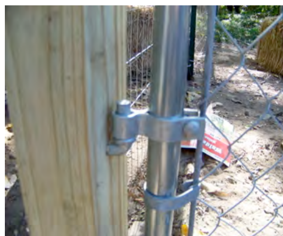
Figure 36. Bottom lag screw with hinge
