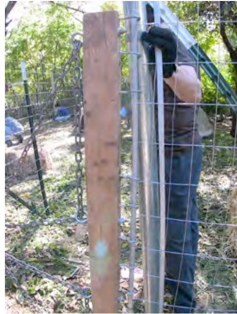
Figure 22. Attach fence-puller to tension bar
