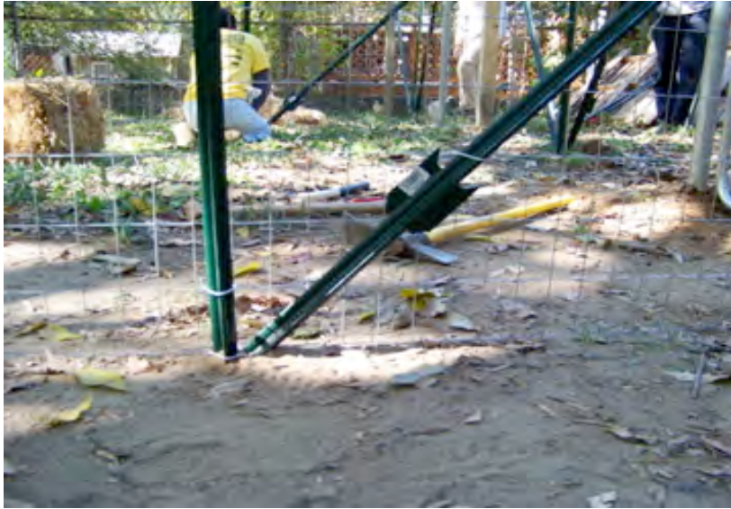
Figure 9. Diagonal support against vertical t-post
