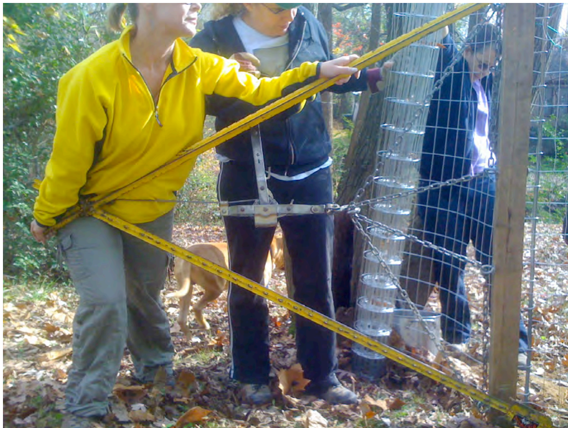
Figure 25. Crank the come-along to tighten the welded wire
