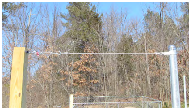
Figure 10d. Finished turnbuckle assembly
