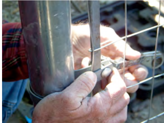
Figure 29. Secure the tension rod to the metal post
