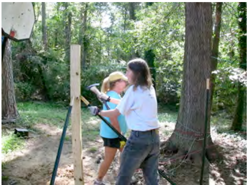
Figure 7a. Hammer the diagonal support into the corner post.
