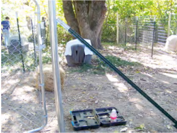
Figures 11a and 12. Diagonal support secured to metal gate post.
