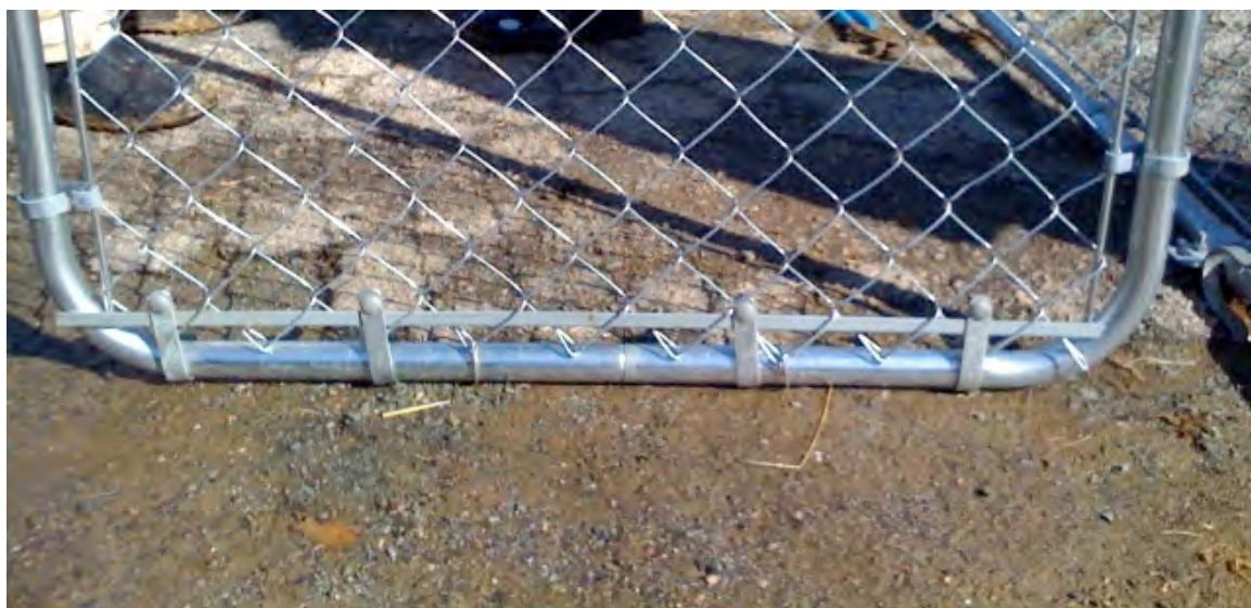
Figure 33. Tension bar and small tension bands to reinforce bottom of the gate.
