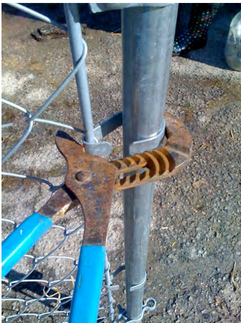
Figure 30: Tightening the tension hooks
